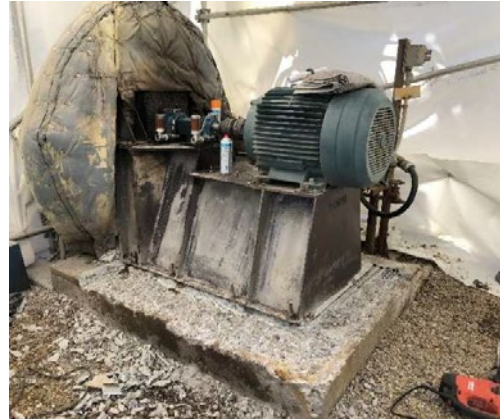
Figure 13: In-Process of Removal of Existing Epoxy Grout and Underlying Concrete
