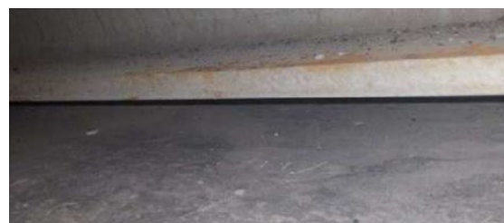
Figure 8 - Unsupported Areas due to poor grouting under the skid
