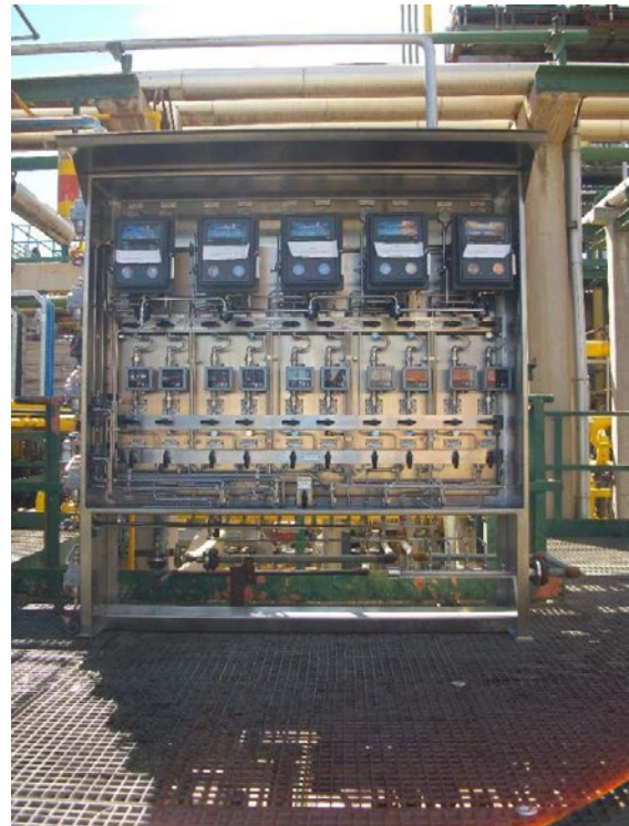
Figure 10: Vent monitoring and buffer gas control panel for compressor unit 2
