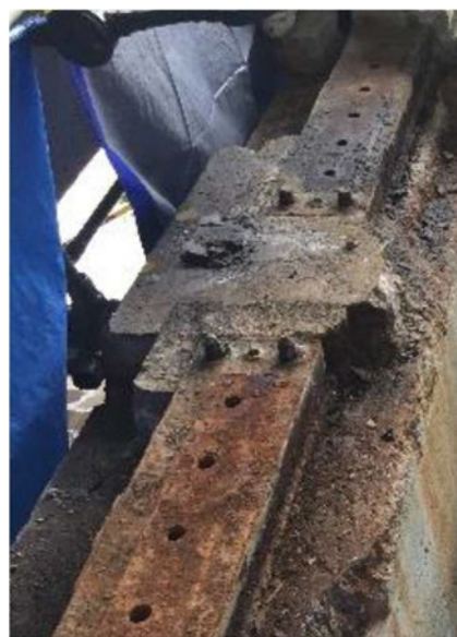
Figure 2: Removal of Existing Cementitious Grout
