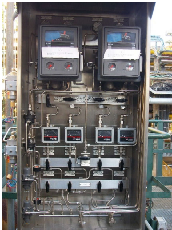
Figure 9: Vent monitoring and buffer gas control panel for compressor unit 1
