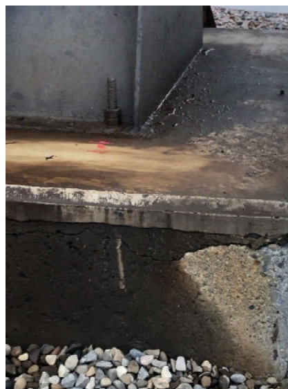
Figure 11: Edge Lifting on Foundation
