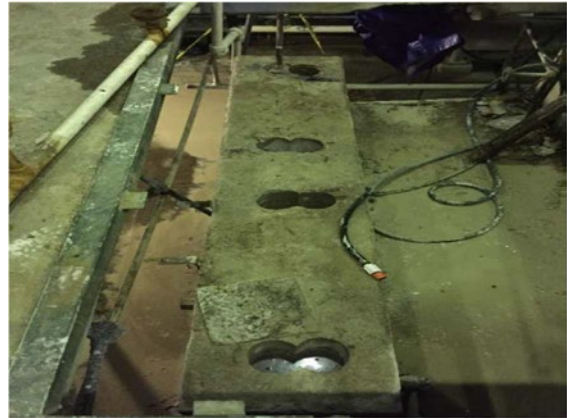
Figure 6: Foundation After Damaged Anchor Bolts Removed
