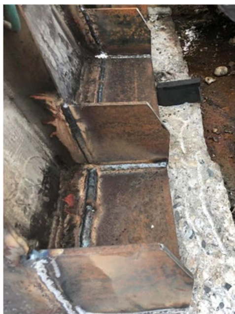
Figure 15: Baseplate Extension Welded to Existing Baseplate
