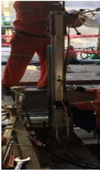
Figure 5: Core Drilling Damaged Anchor Bolts
