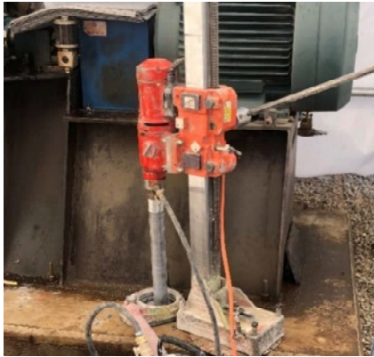
Figure 12: Core Drilling New Anchor Bolt Pockets
