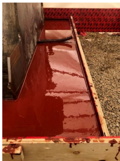
Figure 17: Superior Epoxy Grout Installed in New Anchor Bolt Pockets and Under Baseplate and Baseplate Extension
