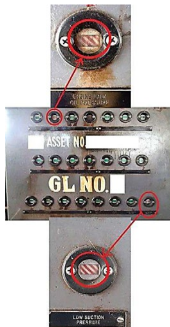
Figure 8: An example of Unit trip reason ambiguity in our pneumatic panels
