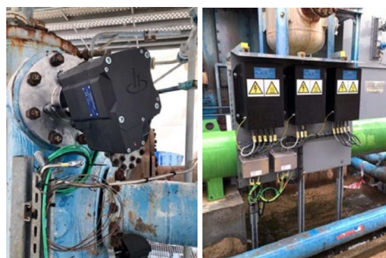
Figure 7: (Left) New electric actuator installed on a valve cover, and (right) the three FPSUs mounted alongside the compressor.
