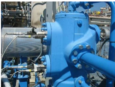
Figure 3: Pressure transmitters and Kiene valves.
