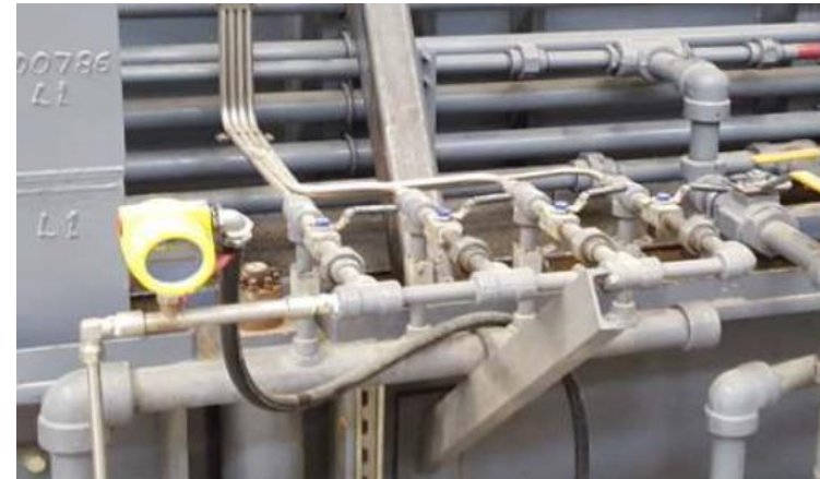
Field installation of individual vent flow lines for each cylinder (GMRC 2016 Atmos Energy)
