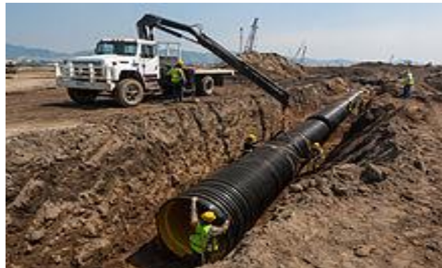
HDPE pipe installation in storm drain project in Mexico
