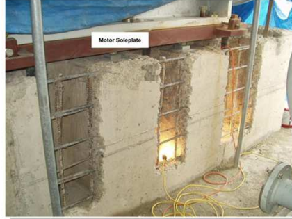
anchor bolt position was off
