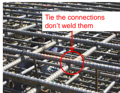
Reinforcement Matrix Showing Tied Connections (source GMRC)
