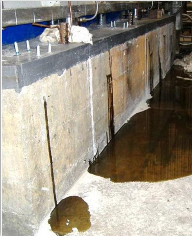
Foundation Crack Repair by High Pressure Epoxy Injection
