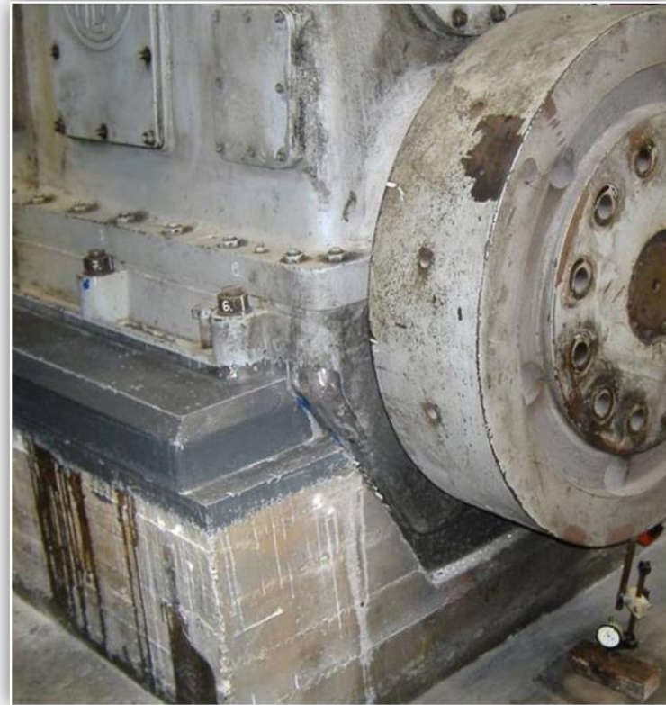
Refurbished Foundation with new Epoxy Grouting – Fit for Purpose
