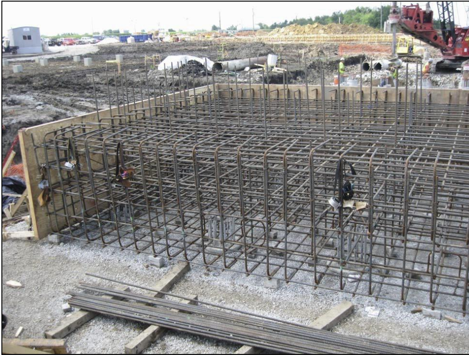
Foundation rebar matrix for anchor bolts (source GMRC)
