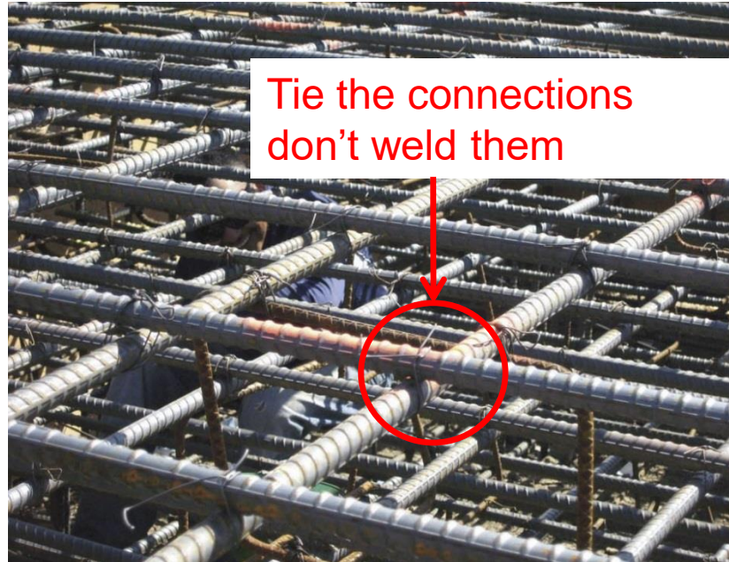
Reinforcement Matrix Showing Tied Connections (source GMRC)
