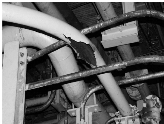
Figure 2: Torn safety valve inflow pipe of the 5th stage
