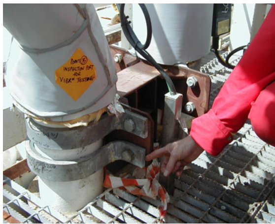
Figure 10: Photo of a part of the system with a loose clamp
