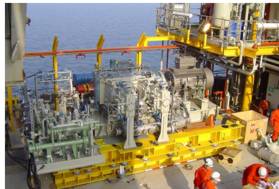
Figure 13: Compressor package on site
