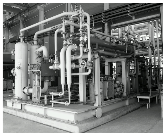
Figure 1: Overview of installation of one hydrogen compressor unit. The location of the local operator console is in the back ground on the right
