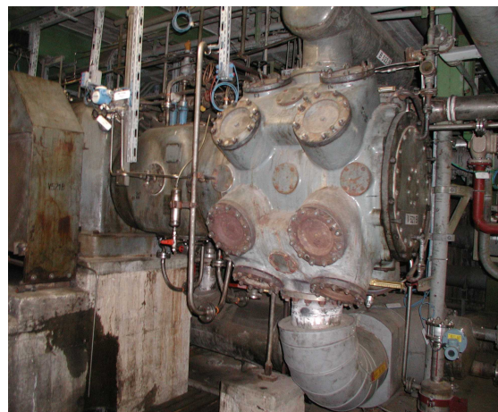
Figure 2: First stage (Ø 620 mm) of the Linde 2-stage piston compressor
