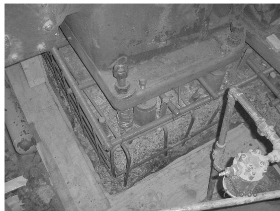
Figure 10: Additional rebar cage installed prior to shuttering
