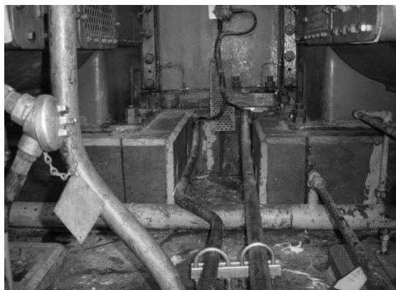
Figure 12: Final grouting installation
