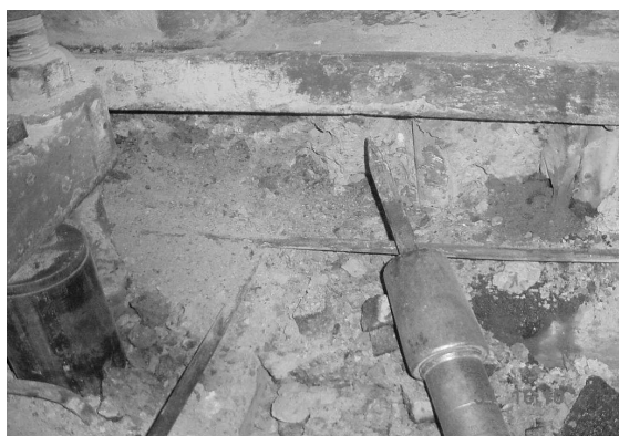
Figure 8: Grouting condition upon breakout showing oil impregnation
