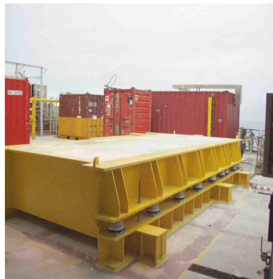
Figure 8: Concrete filled skid, mounted on AVM's
