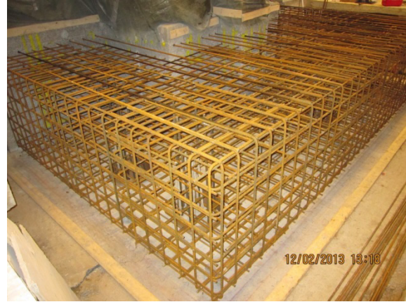
Figure 20: Reinforcement of the foundation extension.
