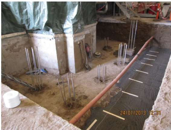
Figure 19: View on one side of the foundation after completion of the concrete piles.
