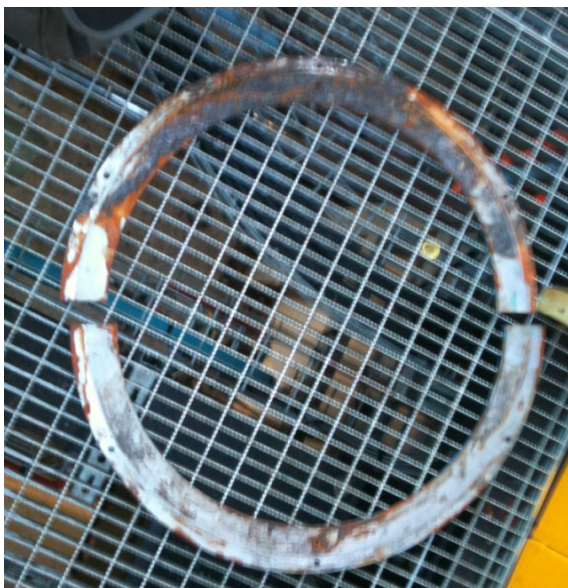
Figure 21: Rusty ring of motor end shaft sealing was found
