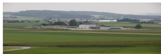
Figure 2: Overview of the Haidach production and storage facilities (UGS Aigelsbrunn and UGS H5)
