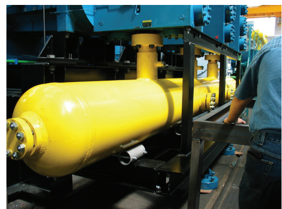
Figure 4 Photo of the discharge 2 nd stage damper
