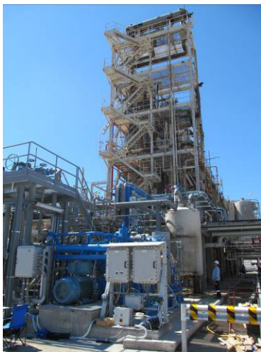
Figure 16: Compressor controlled by Cozzani control system
