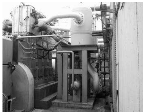
Figure 16: A suction dampener with increased volume was installed with flexible steel piping
