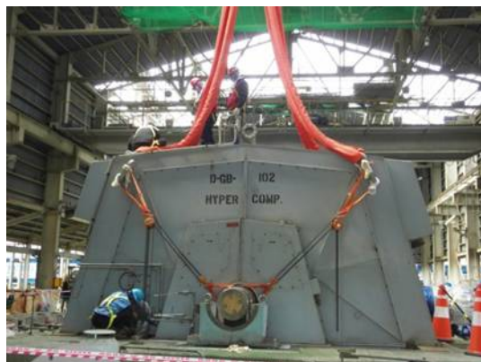
Figure 6: Lifting out existing main driver
