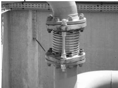
Figure 18: Bad solution for avoiding transfer of vibrations
