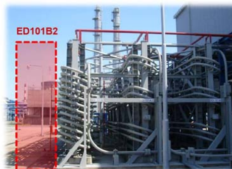
Figure 9: Highlighted area for new intercooler bundle stream "B"
