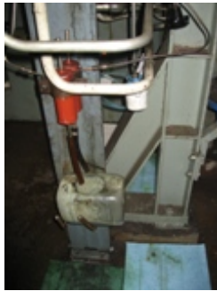
Picture 17+18: Additional Cylinder supports from 1978 delivered by Halberg
