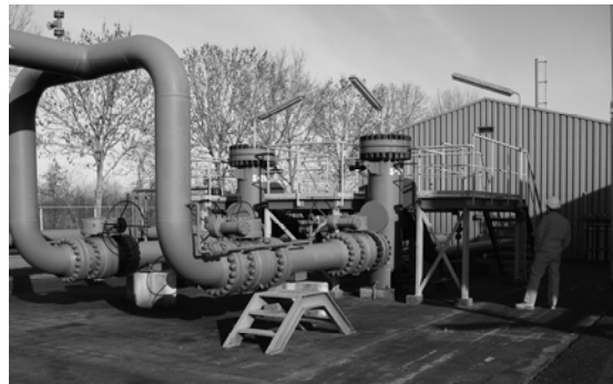
Figure 8: Parallel flow metering streets with filters and flow meter enclosure
