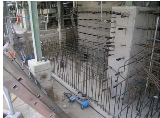
Figure 1: Modification of foundation
