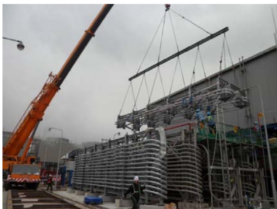
Figure 10: Installation of additional intercooler bundle for stream "A"
