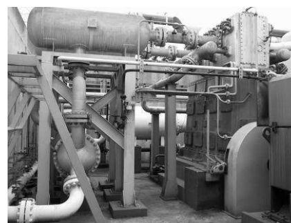
Figure 17: Discharge pulsation dampener in original horizontal position
