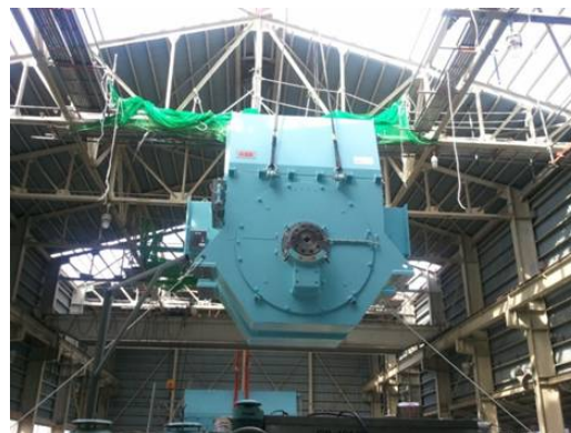
Figure 8: Lifting of main driver through open roof into position
