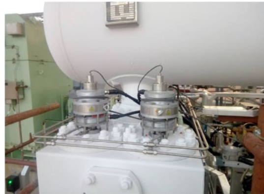
Figure 1. Two actuators of an electromagnetic capacity control system.
