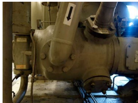
Figure 6: The first and third stage cylinder.
