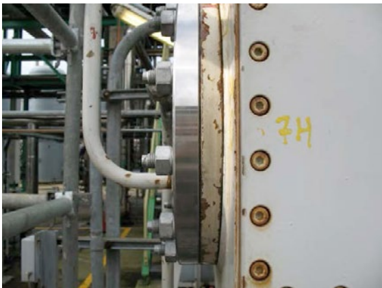
Picture 5: Side view of new reinforcement ring and studs after installation on the head
