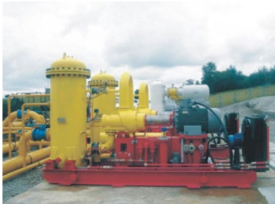
Fig. 6 Equipment for natural gas compression, containing screw compressor (Source: Comoti 2 )
