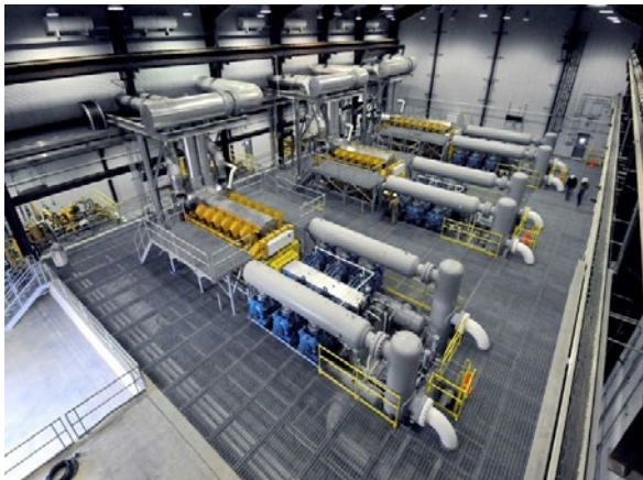
Figure 1: Multiple 6 MW compressor packages used in natural gas transmission service.
