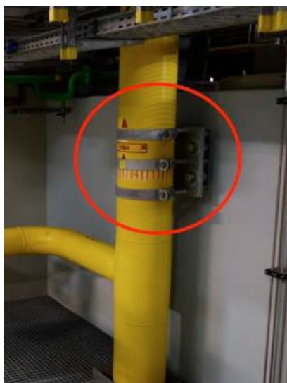
Figure 14 Recommended additional pipe support
