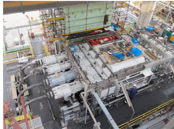
Figure 1: K8 Hyper compressor with the monitored cylinder in gray color on the left hand side.
