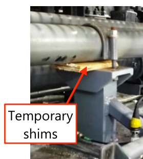
Figure 4.4 – Temporary shims under the pipe
