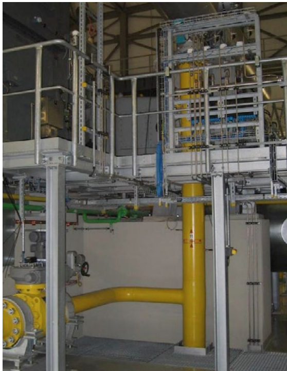
Figure 3 Vertical inlet pipe of the suction 1st stage
