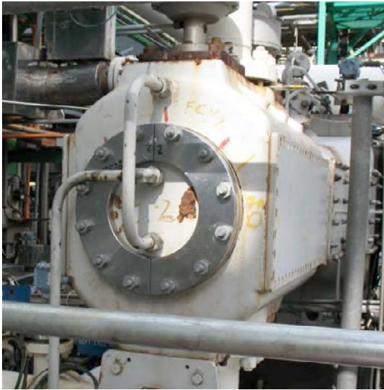
Picture 4: Front view of new reinforcement ring and studs after installation on the head
