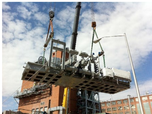
Figure 10: Compressor package installation at a U.S. chemical plant
