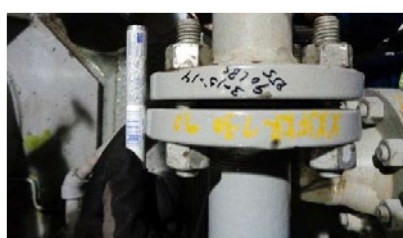
Figure 4.5 – Flange misalignment
