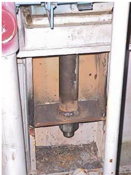
Figure 11.14 Example of achieving extended length of crosshead guide anchor bolts with reinforcing horizontal plate [6]
