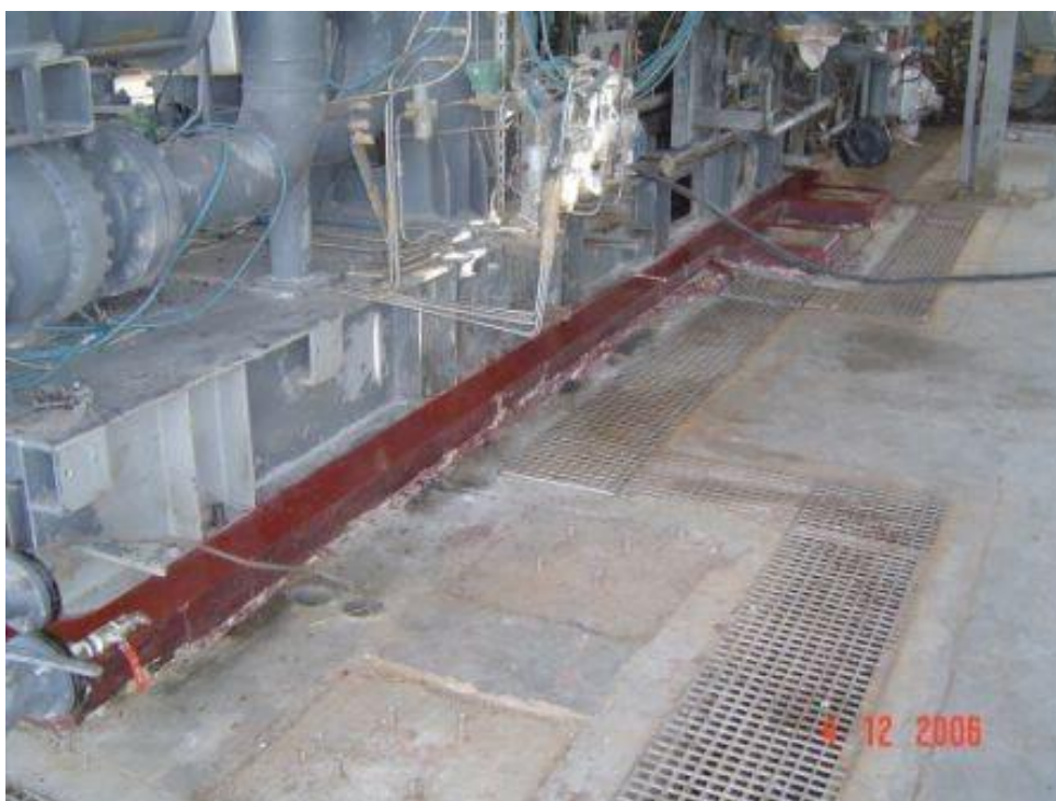
Figure 12.8 Example of a full bed grouted skid [14]
