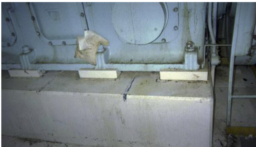
Figure 12.14 Example of a poured in place chocks [20]
