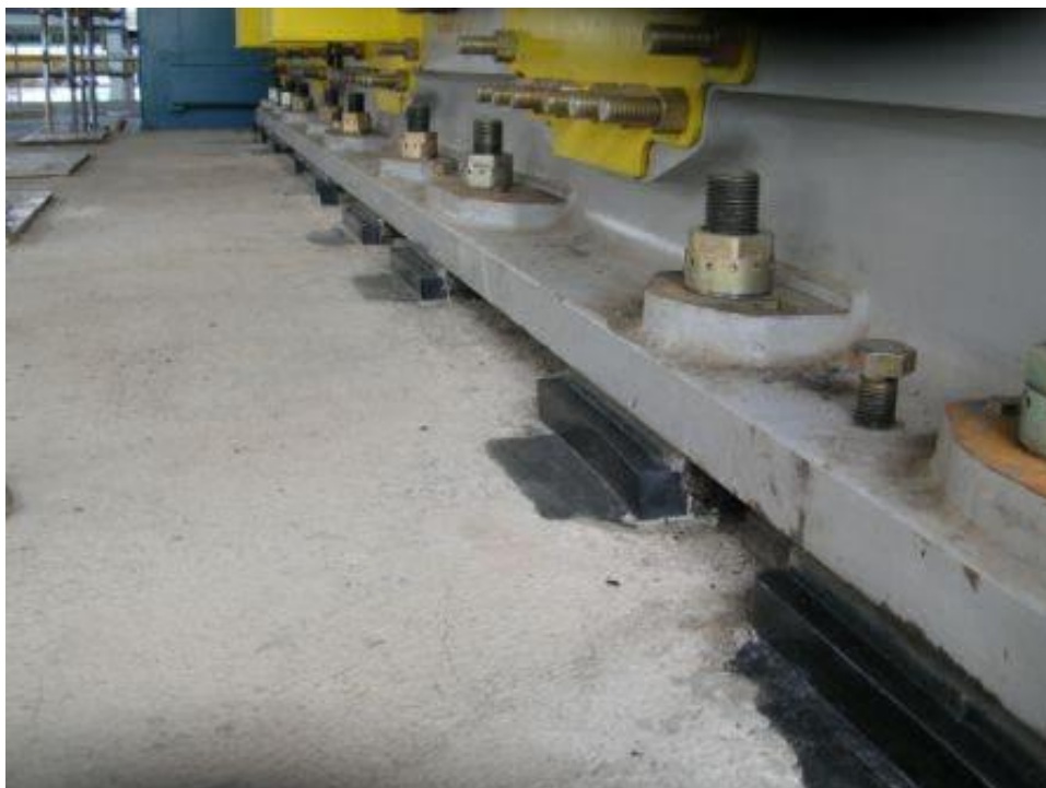
Figure 12.7 Example of a skid mounted with shims and epoxy chocks direct to concrete block [14]
