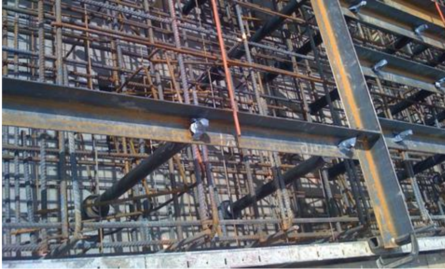
Figure 8.1 Example of a steel anchor bolt template plate (pre-installed)
