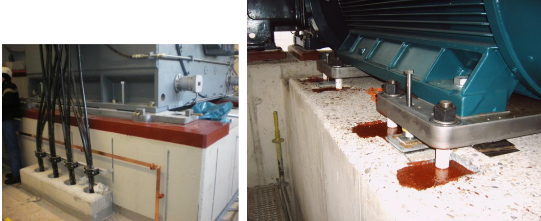
Figure 13.2 Mounting examples of an electric motor with shims and soleplates in grout bed [14]
