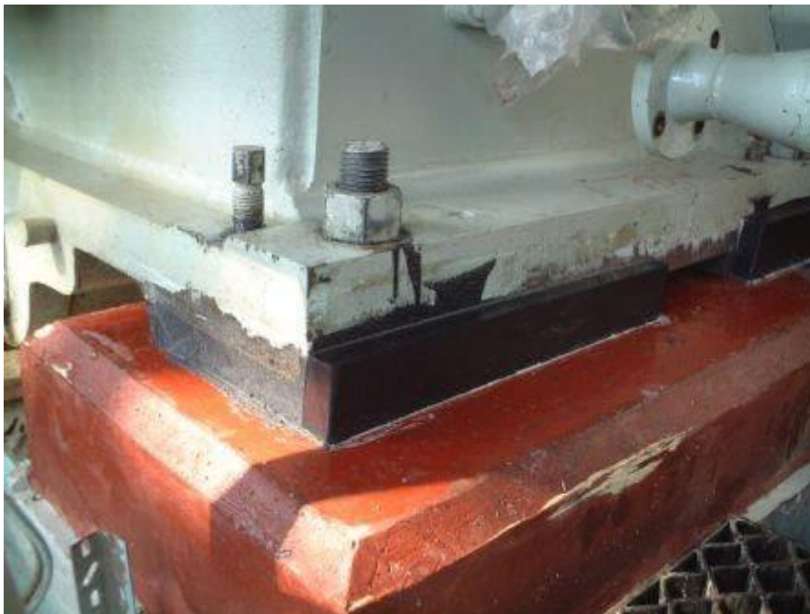
Figure 12.5 Example of compressor mounted with grouted sole plates and grouted chocks to concrete [14]
