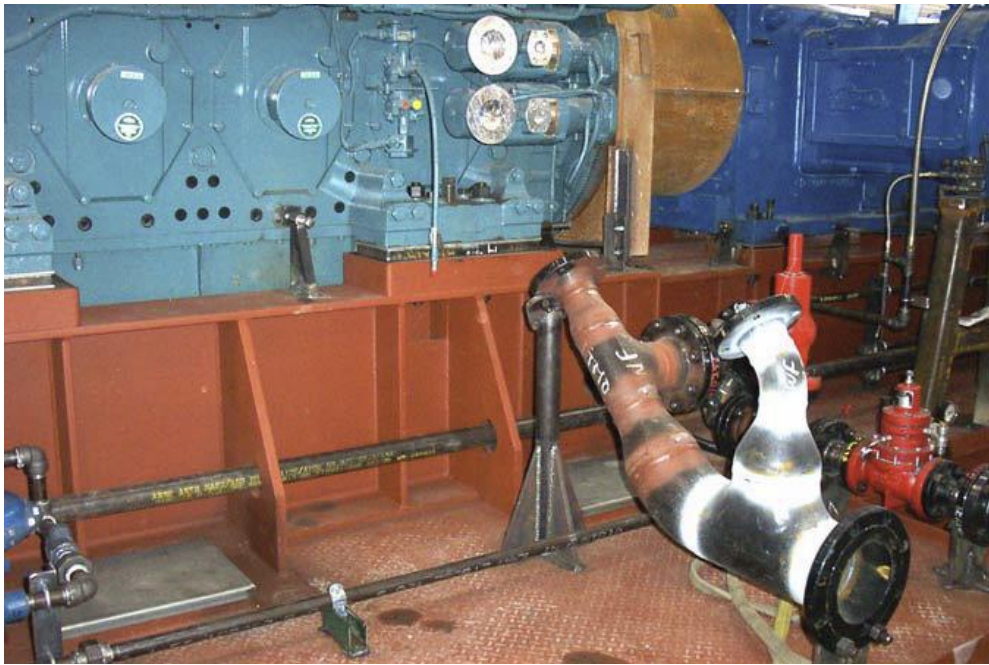
Figure 13.1 Note engine foot mounted via shims on chock set in “red” grout box. Grout box is welded to skid. Note heavy gusseting of skid [6]
