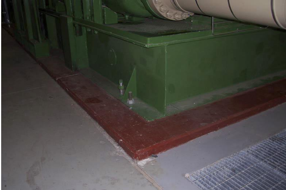
Figure 12.9 Example of a full bed grouted skid [14]
